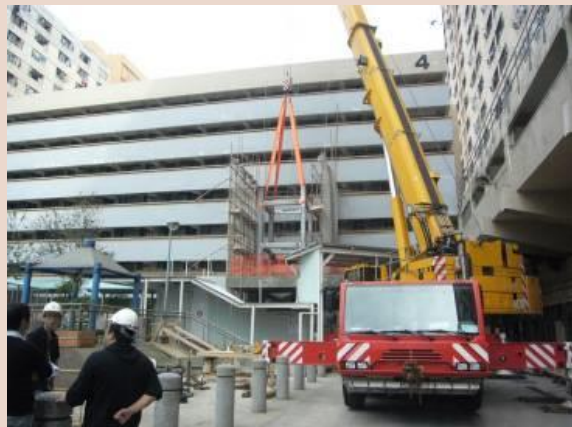
STEEL FRAME INSTALLATION
