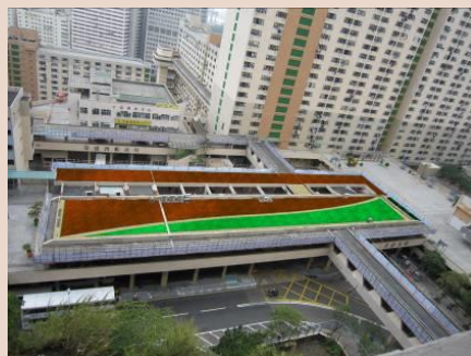
Green Roof and Vertical Greening
